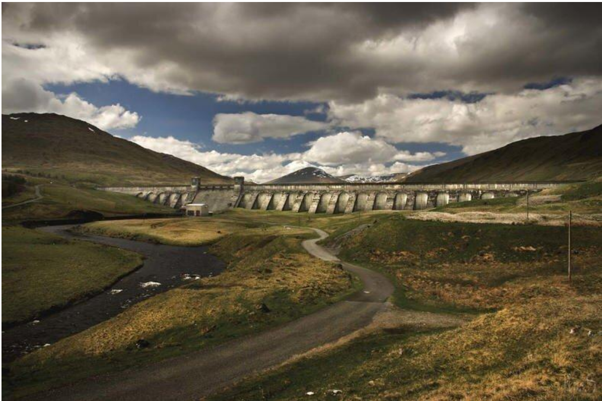
Lubreoch Dam and Power Station, Glen Lyon
